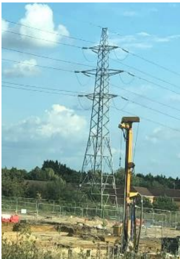
Figure 9 132kV Tower Mounted Overhead Power Lines
