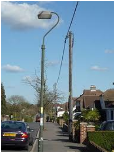
Figure 1 Aerial Bundle Conductor Low Voltage Overhead Power Lines
